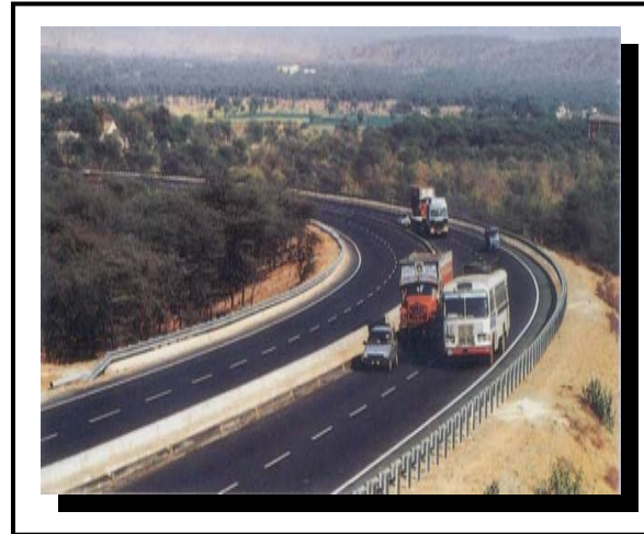
New highway infrastructure
